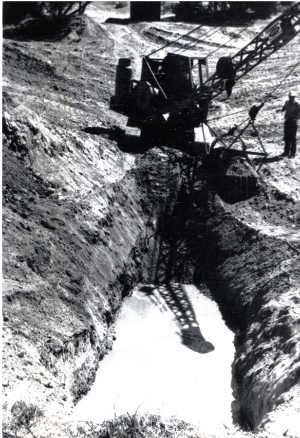
Initial cut, west end of trench.
