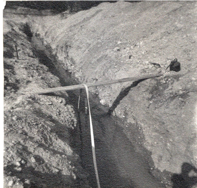
Result of trying to relocate discharge hole (hose leads to pump).
