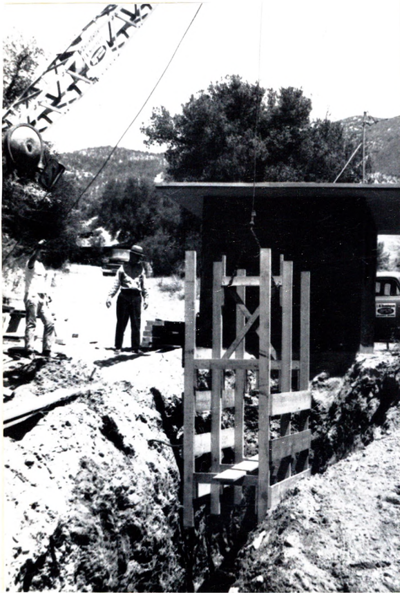
Dragline lowering timberset into cutoff trench.
