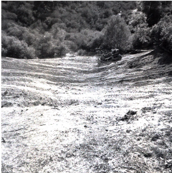
Partially cleared trench site from pump house.
