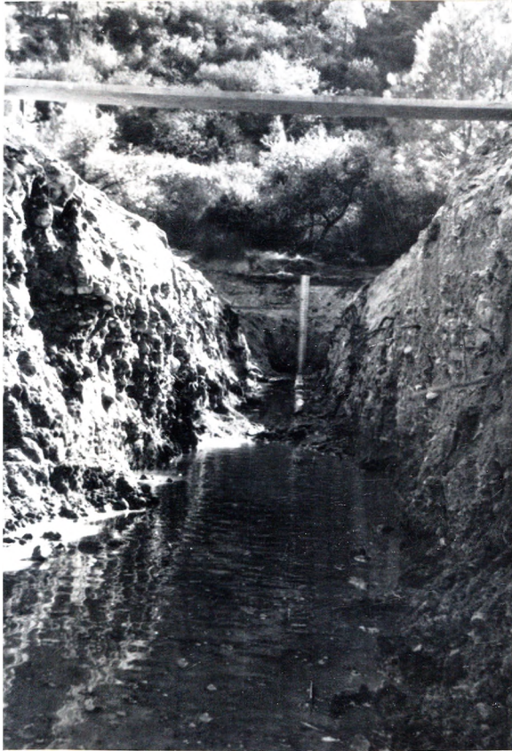
Lamp-hole installed at west end of trench.
