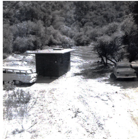
Pump house with trench site in background.
