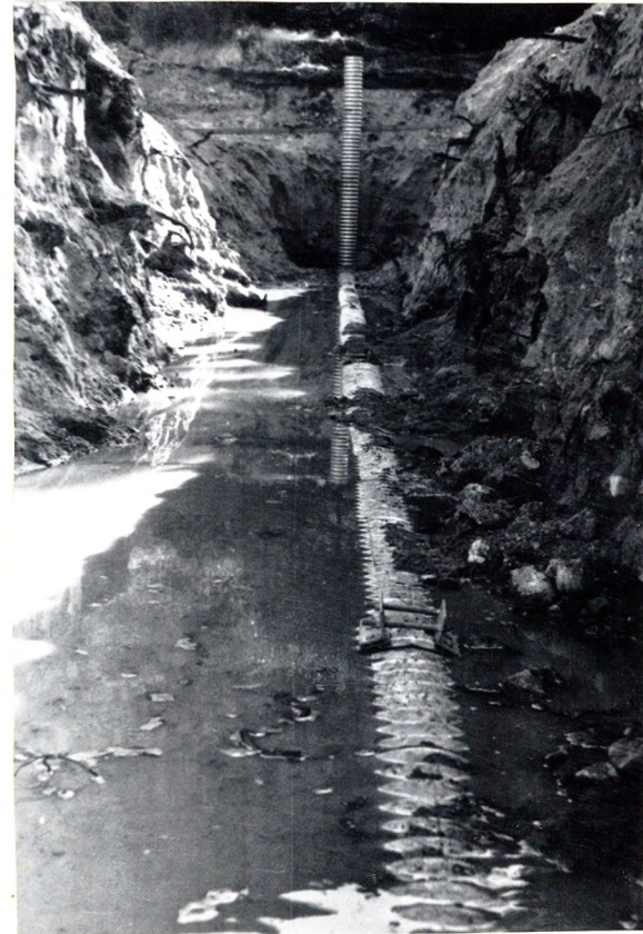
Perforated pipe in bottom of tunnel.
