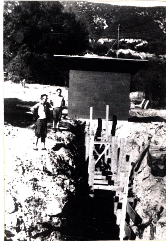
Installed timber set.
